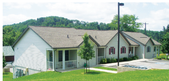
Campbell Place (top) and Independence Gardens (bottom) are a pair of Cambria County, PA, affordable housing renovation projects that FNB supported through its FHLB membership.
